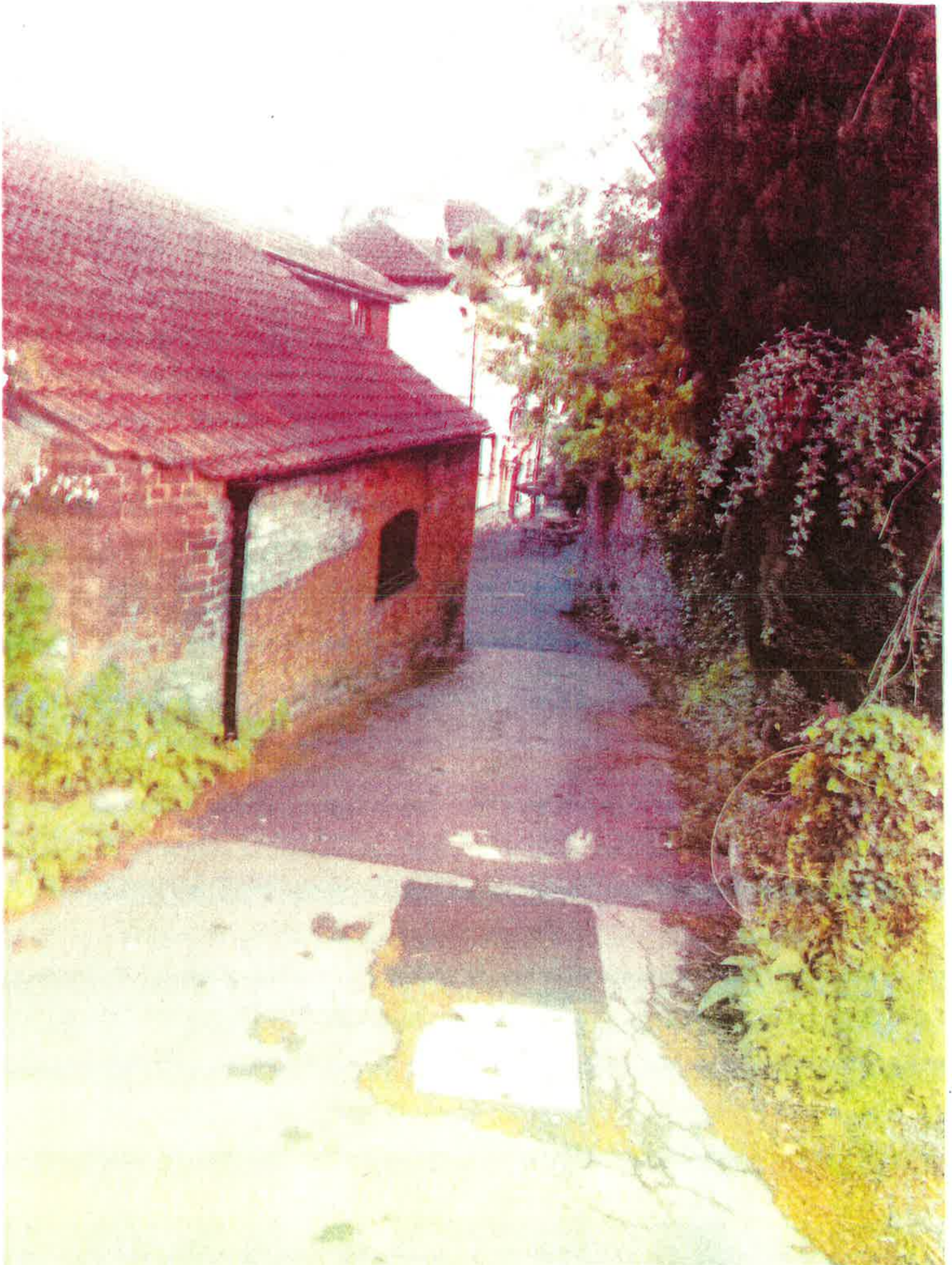
Breach of condition - dated, 06/06/2013
